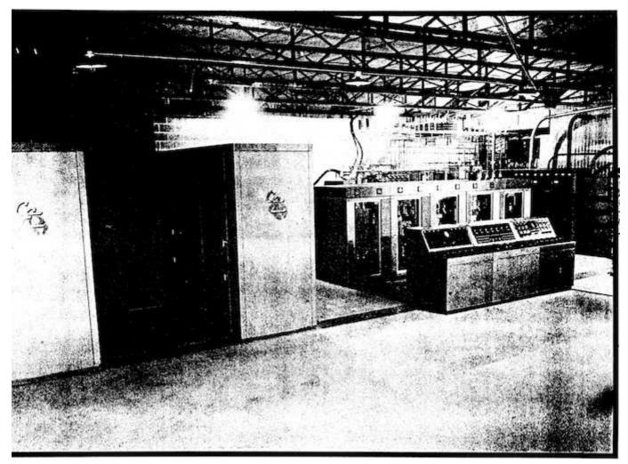
The Type 420A transmitter has been designed for AM operation in the International Shortwave Broadcast Band from 5.9 to 21.75 megacycles with an output power of 500,000 watts carrier, to which modulation of 100% may be applied.
